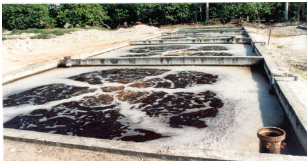
Kolam Aerobik ( completely mixed aeration )
