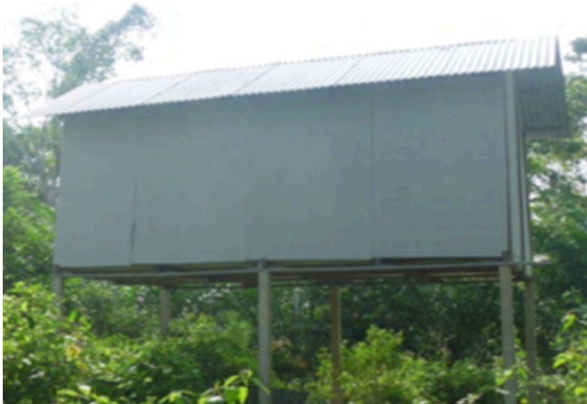
Figure 4. A Swiftlet house in Pahang using Gable Roof design. Cement boards are used for wall and plywood for floor.
