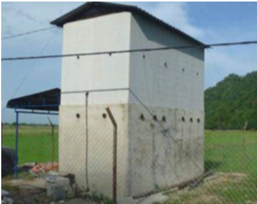
Figure 3. A Swiftlet house in Perlis using Gable Roof design and cement board as the wall and floor.
